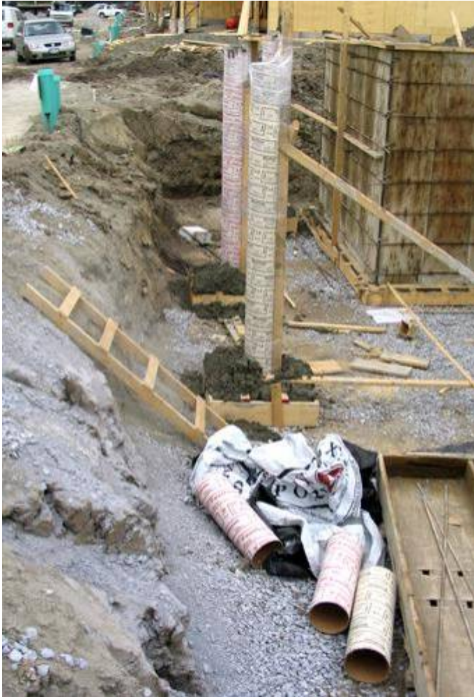
Figure A1b: Commercially available conventional cardboard formworks on a job...
