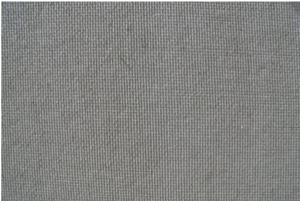
Figure 1: Close up view of the texture of a fabric formed concrete wall.
