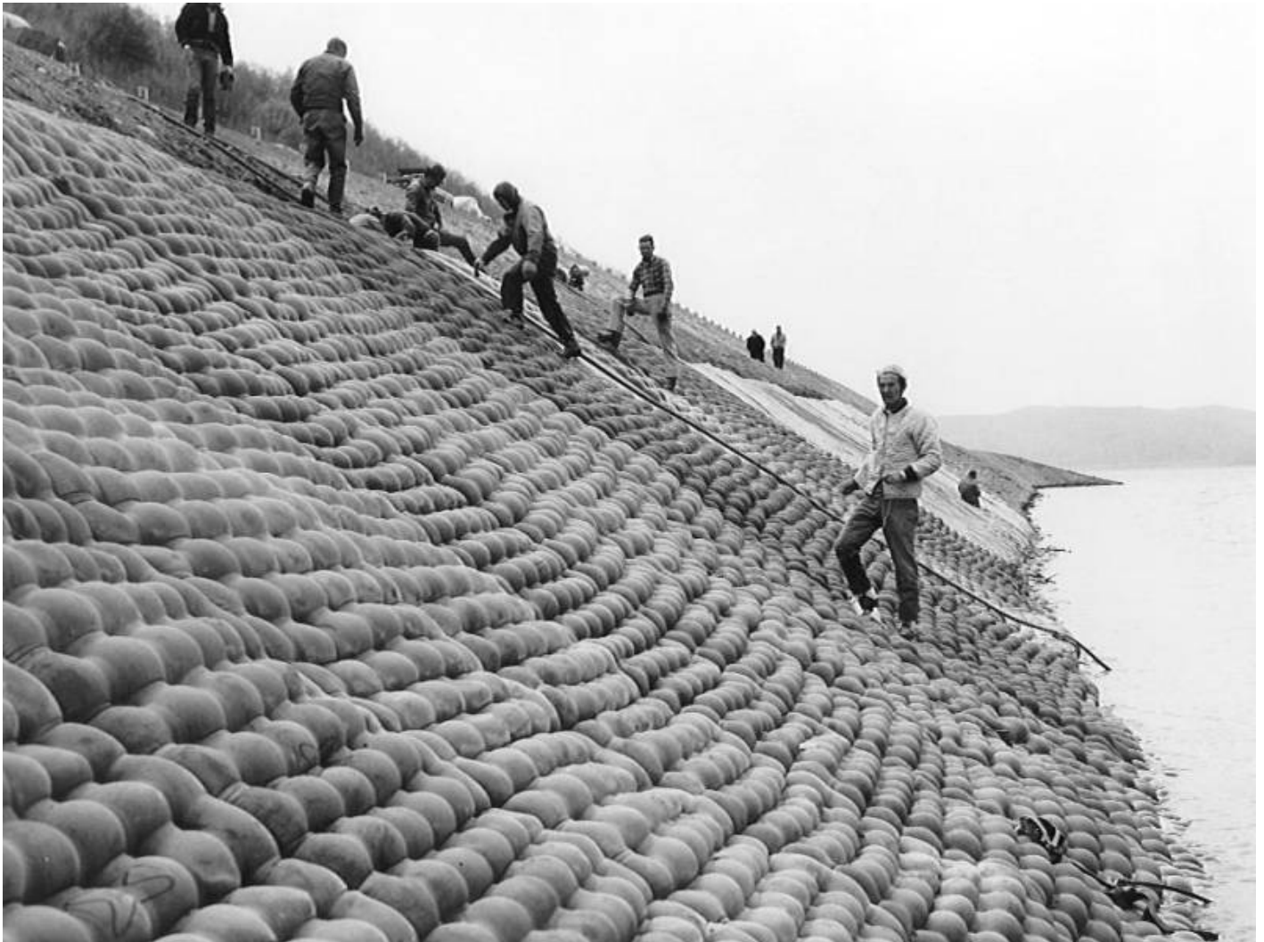
Figure 5: River bank stabilization bags (Fabriform) installed in 1967 on the...
