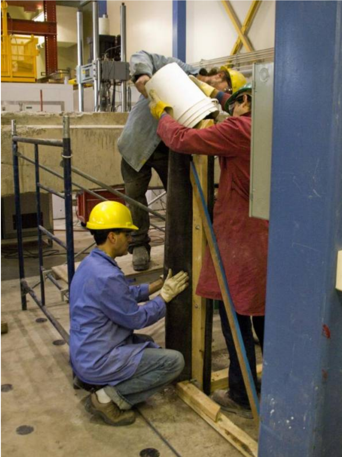
Figure 47: casting of column in fabric formwork.
