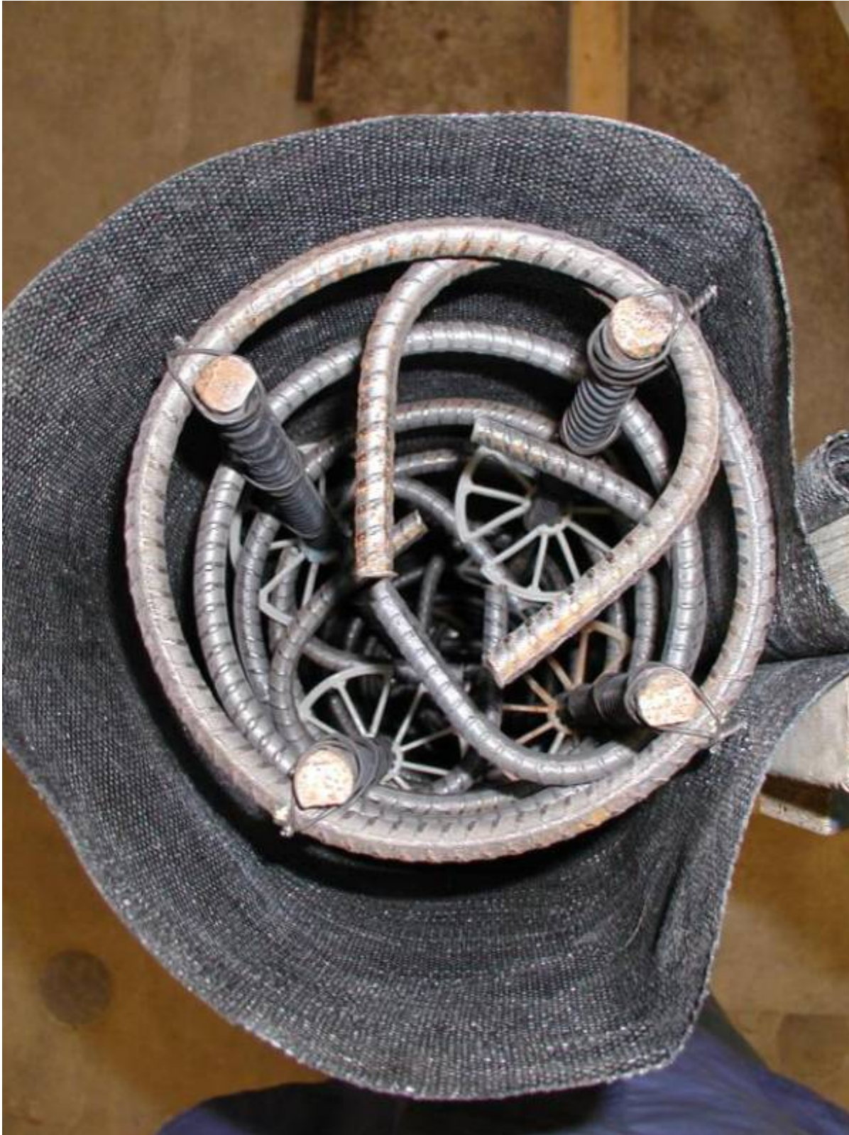
Figure 46: Reinforcement cage.
