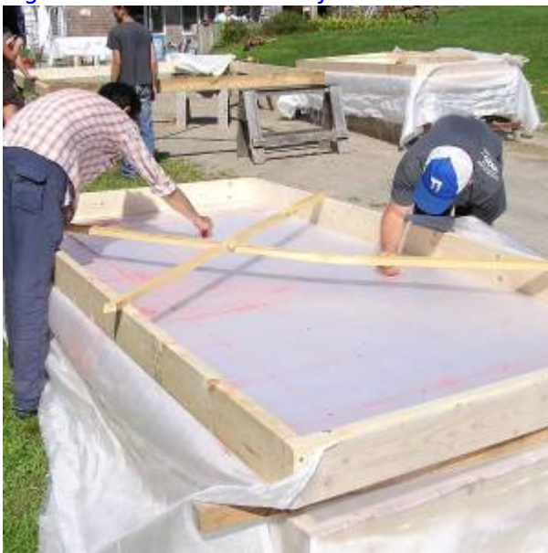
Fig. 3. Wall Form Assembly
