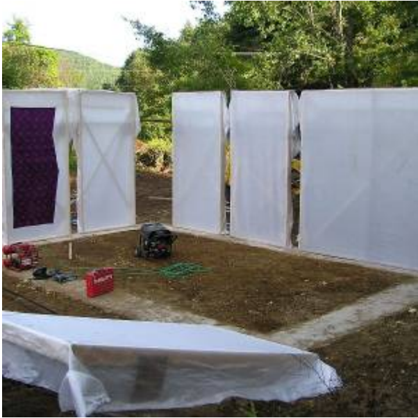
Fig. 4. Wall Form Placement
