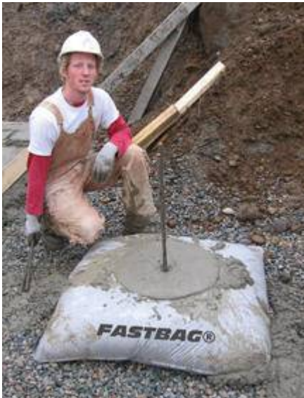
Fig. 3. Spread Footing Application
