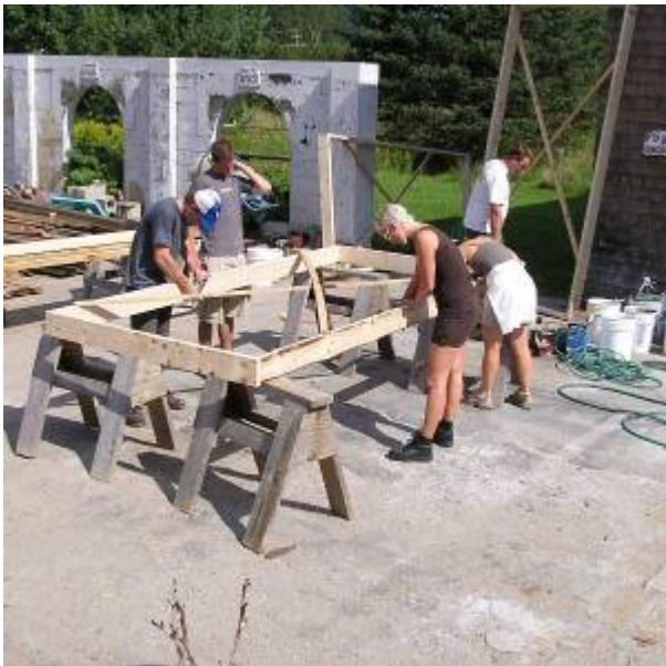
Fig. 1. Wall Form Assembly
