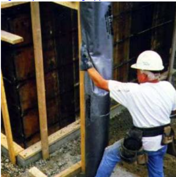
Fig. 4. Spread Footing Application
