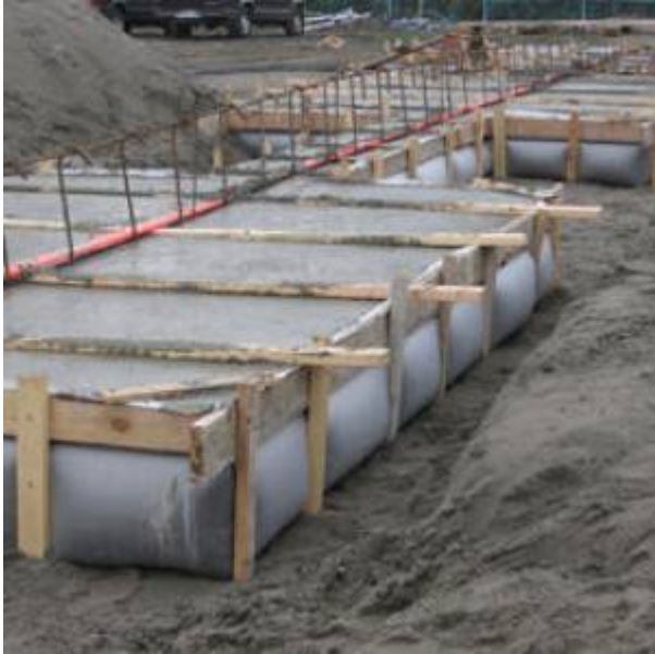
Fig. 2. Spread/Continuous Footing Application
