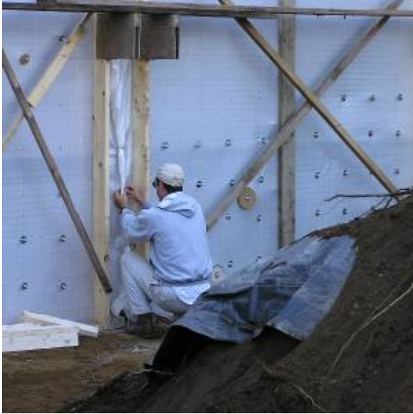
Fig. 7. Wall Form Placement
