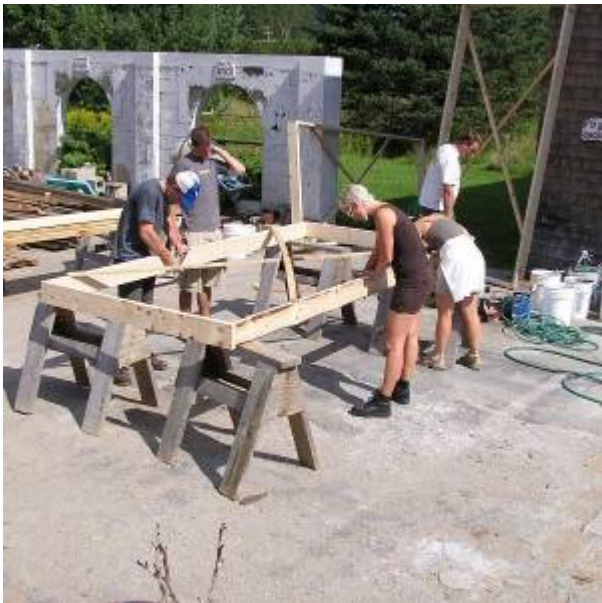
Fig. 1. Wall Form Assembly
