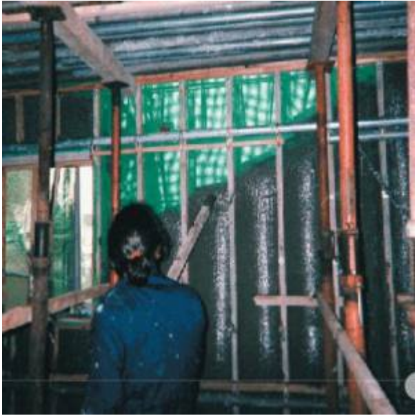
Fig. 1. Frame Form Method
