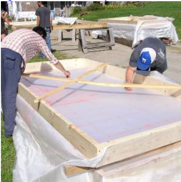
Fig. 3. Wall Form Assembly
