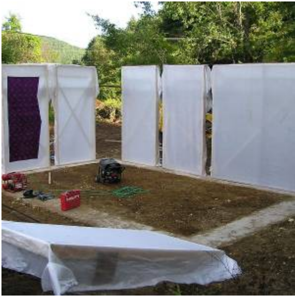
Fig. 4. Wall Form Placement
