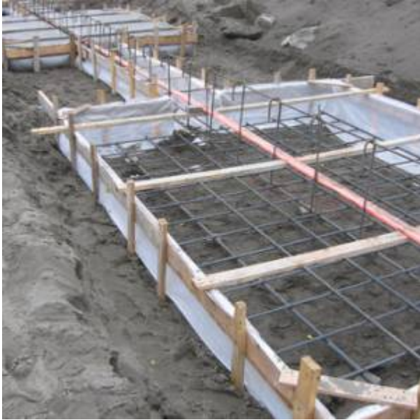
Fig. 1. Spread/Continuous Footing Application
