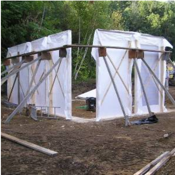
Fig. 5. Wall Form Placement
