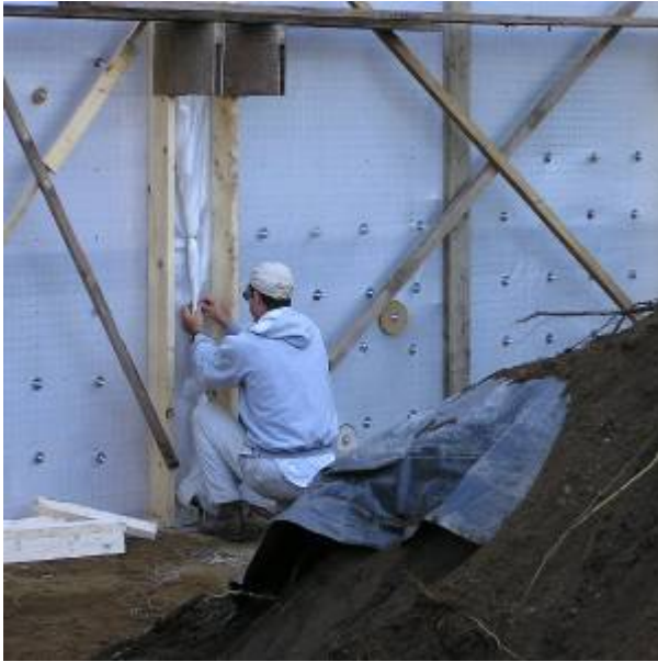
Fig. 7. Wall Form Placement
