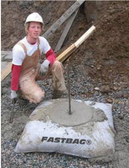
Fig. 3. Spread Footing Application
