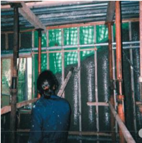
Fig. 1. Frame Form Method
