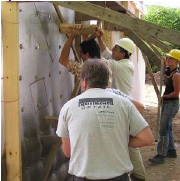
Fig. 11. "Vibrating" Concrete
