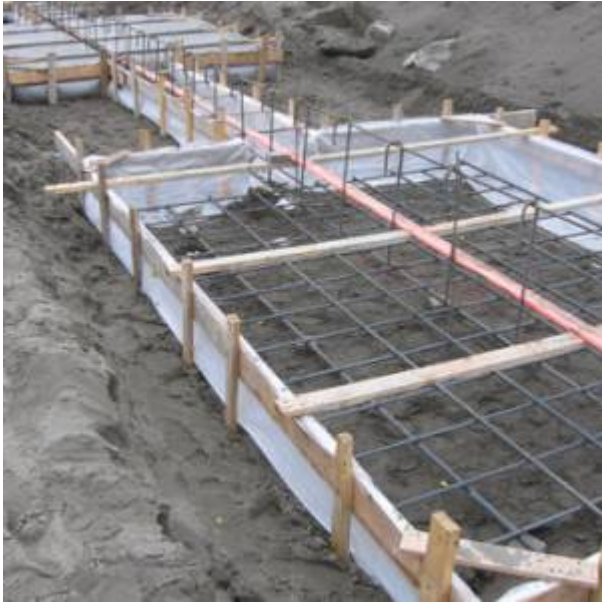
Fig. 1. Spread/Continuous Footing Application
