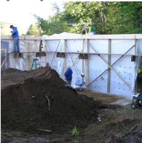
Fig. 7. Wall Form Placement
