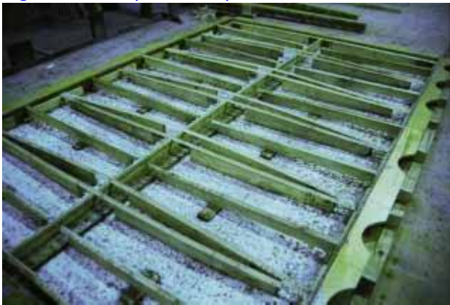
Fig. 9. Formwork for full scale wall panel.
