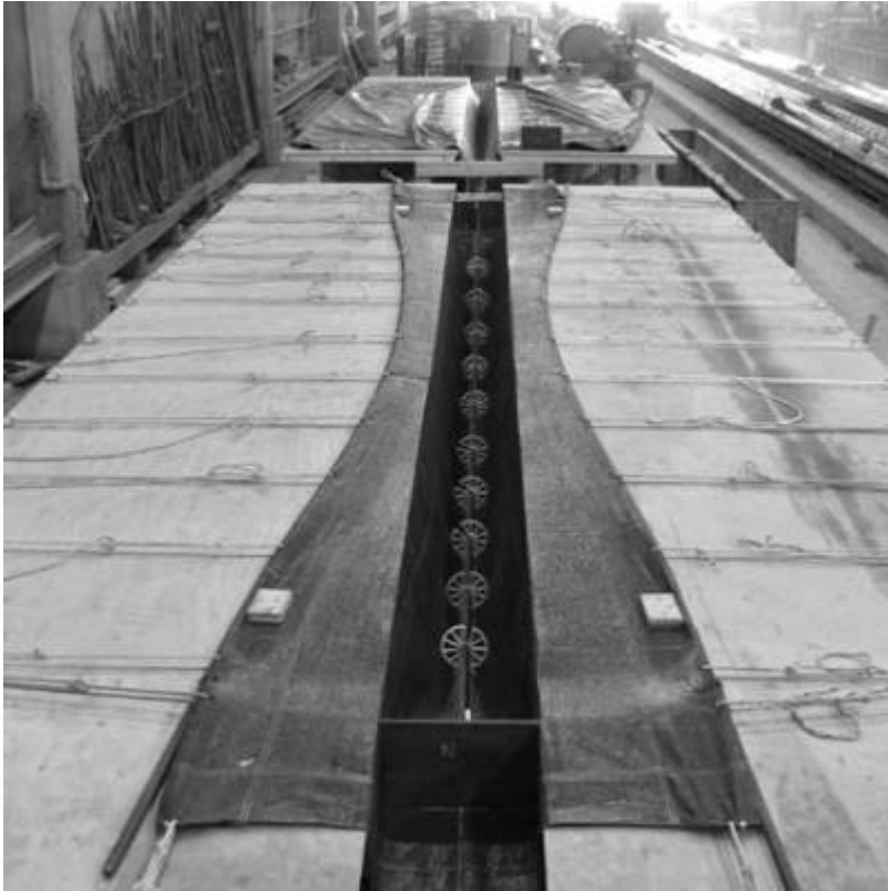
Fig. 5. Plywood deck and fabric formwork for full scale variable section...
