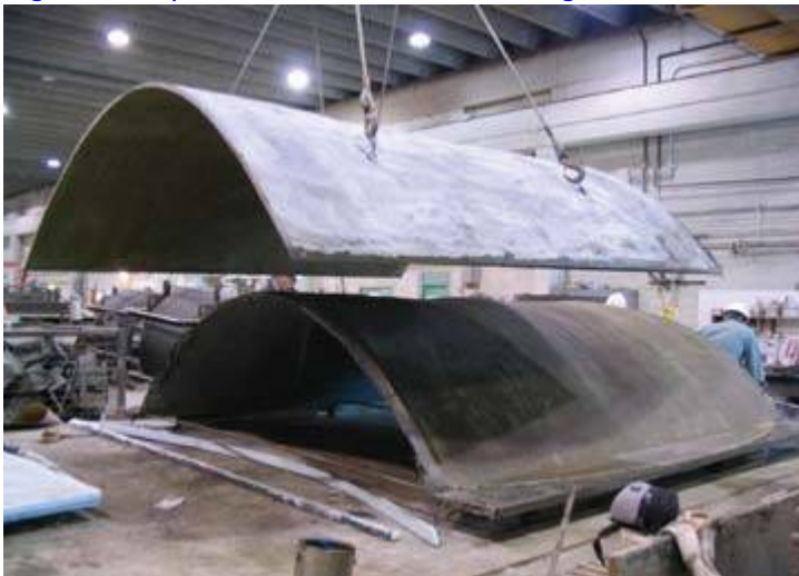
Fig. 23. Step 2- Uniform layer of GFRC is applied.
