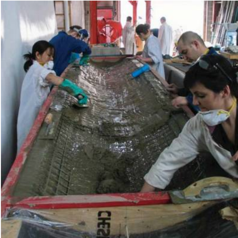
Fig. 34. Placing concrete and carbon grid in fabric mold to form double...
