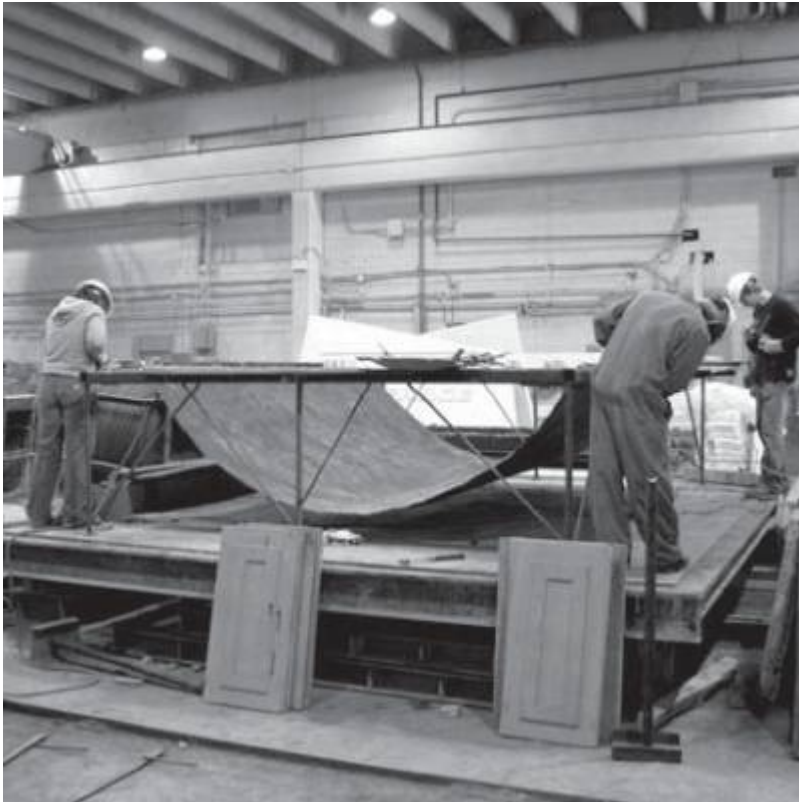
Fig. 22. Step 1 - Geotextile fabric hung from a frame.
