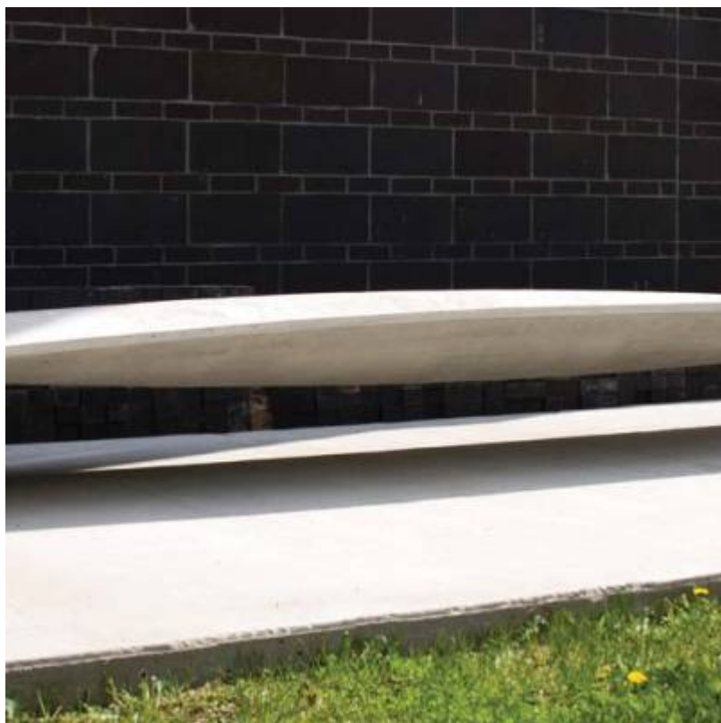
Fig. 41. Completed double-curvature lenticular thin-shell vault.
