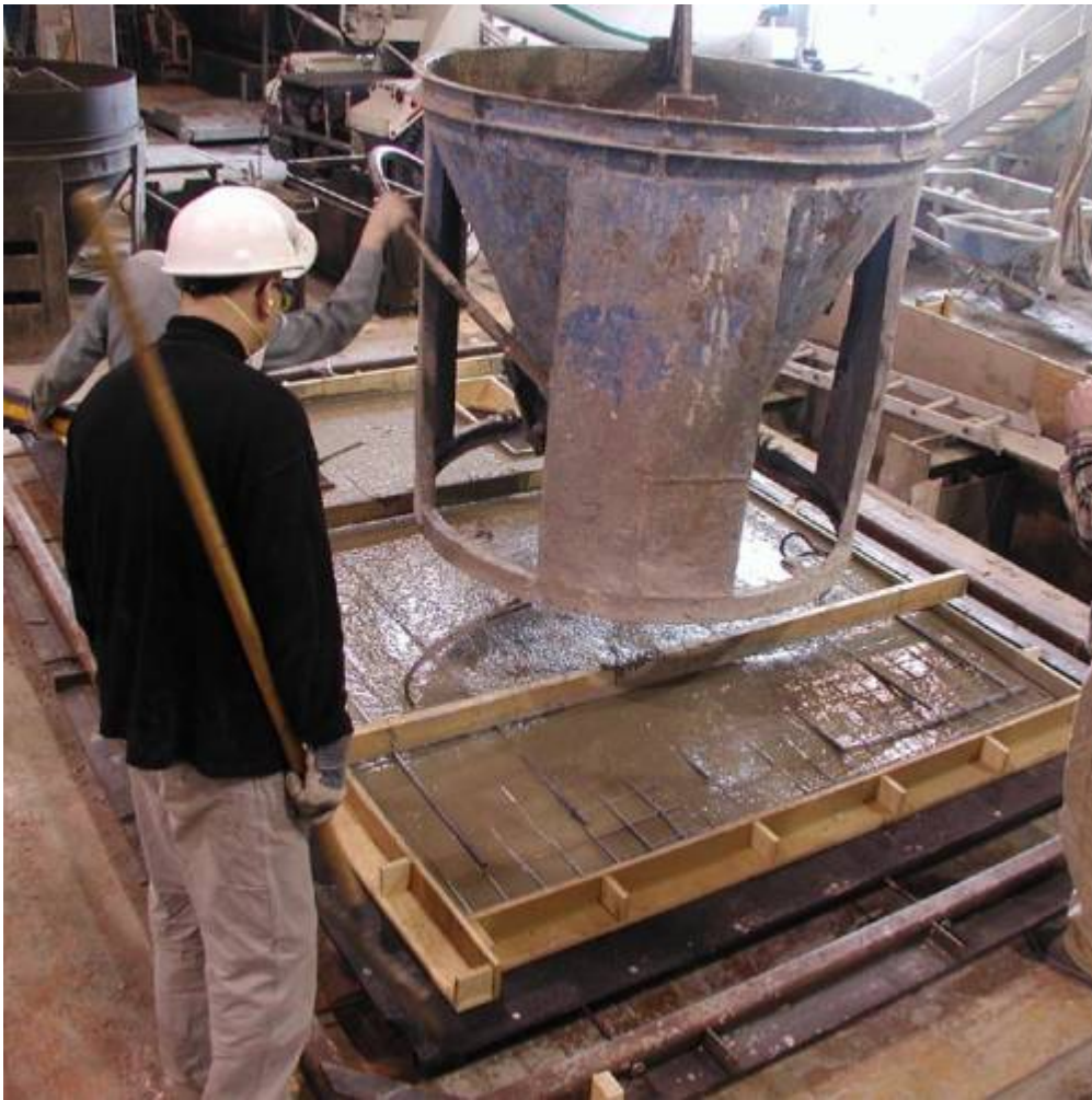
Fig. 6. Placing concrete in full scale wall panel formwork.
