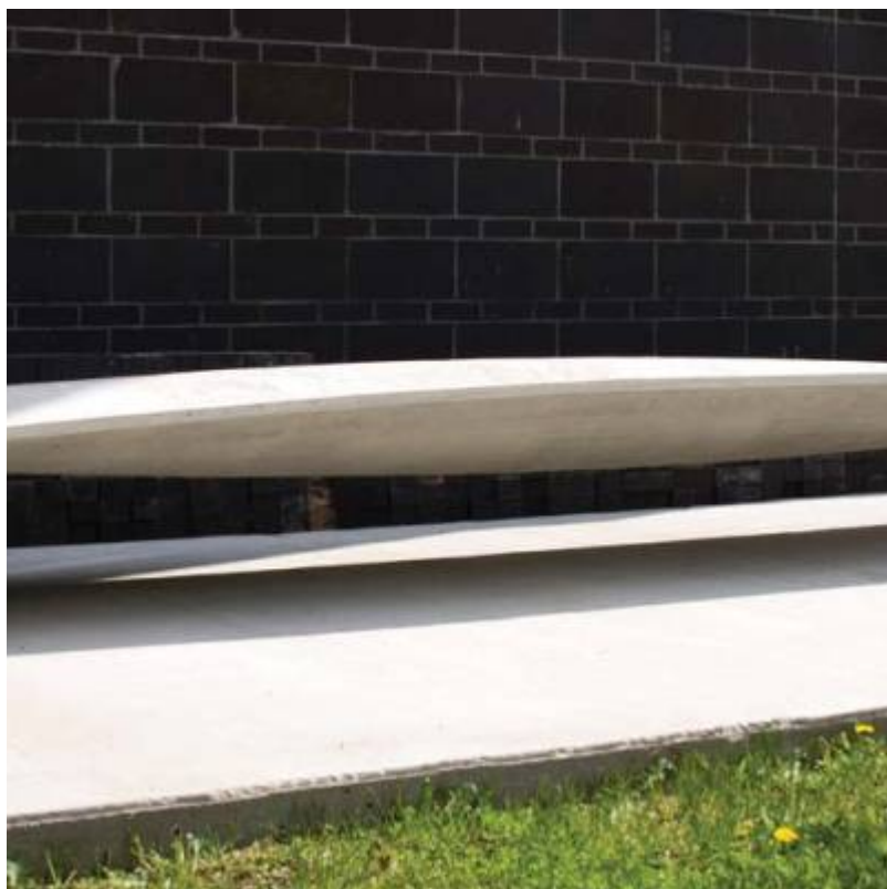
Fig. 41. Completed double-curvature lenticular thin-shell vault.
