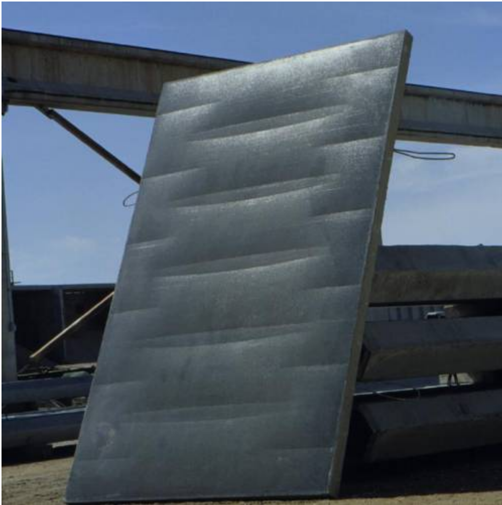
Fig. 10. Completed full scale concrete wall panel.
