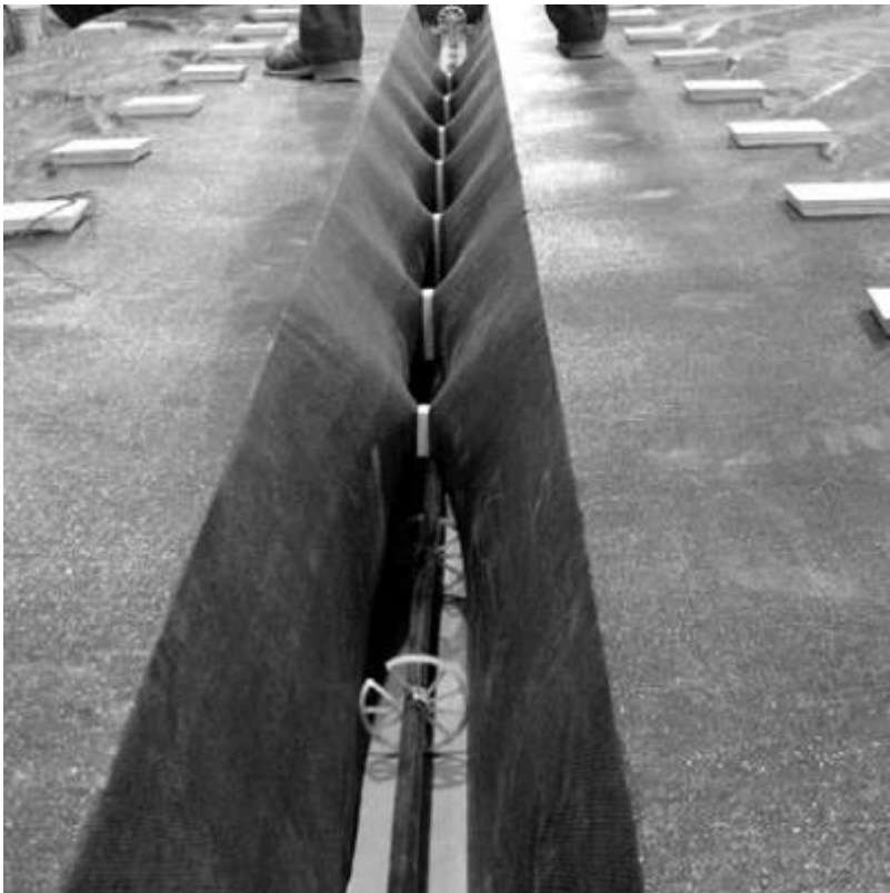
Fig. 7. Fabric formwork for full scale variable section concrete 'pinch'...
