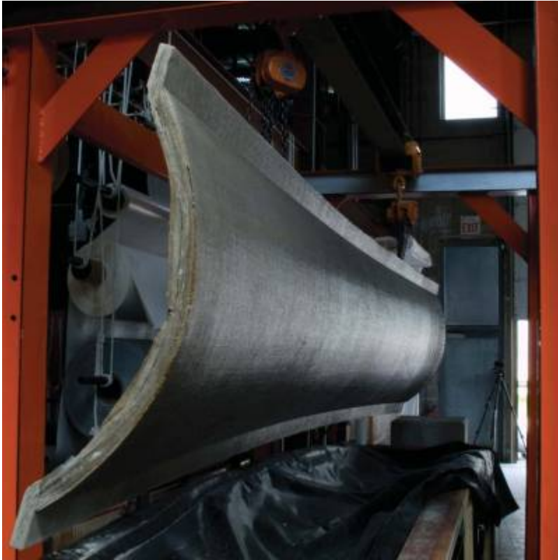
Fig. 35. Removing 3 cm (1.2 in) vault from formwork.
