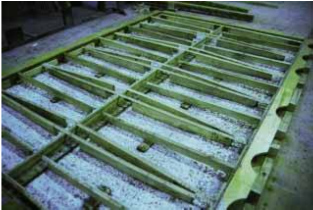
Fig. 9. Formwork for full scale wall panel.
