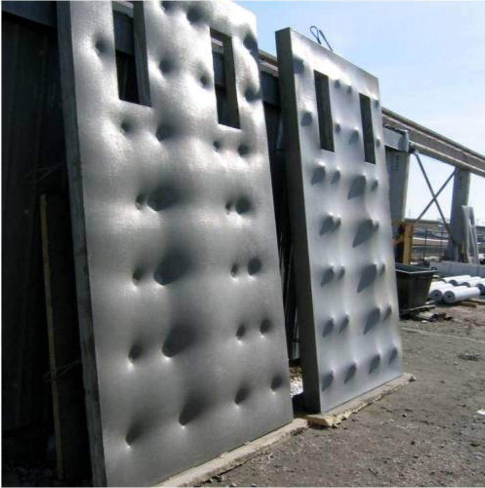
Fig. 7. Completed concrete wall panels.
