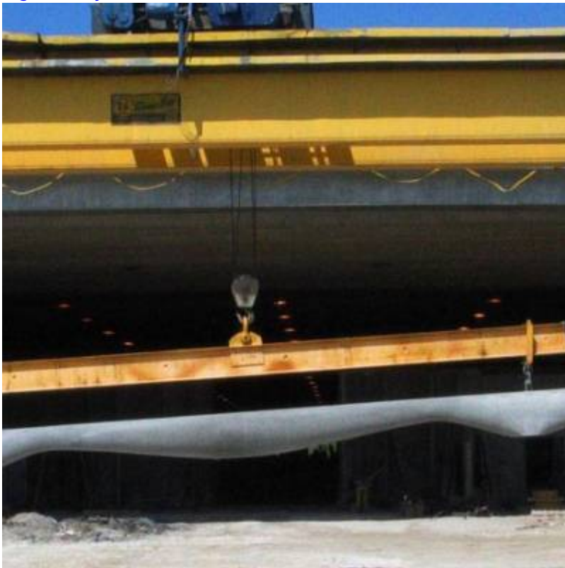
Fig. 12. Completed full scale variable section concrete beam.
