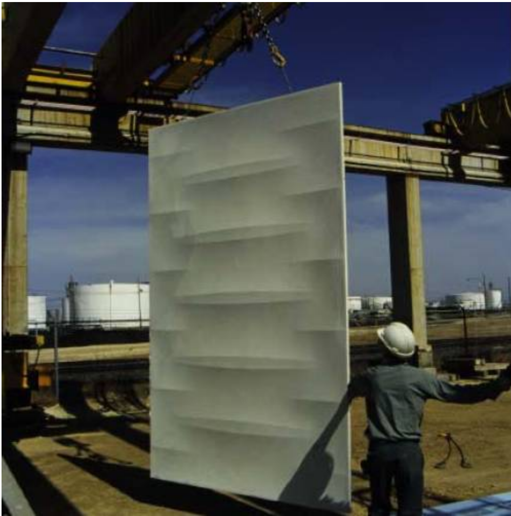
Fig. 11. Completed full scale reverse cast GFRP panel.
