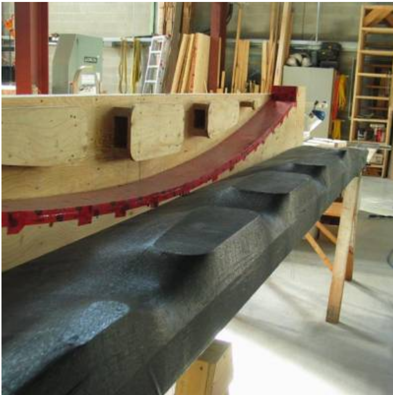
Fig. 3. Model truss formwork.
