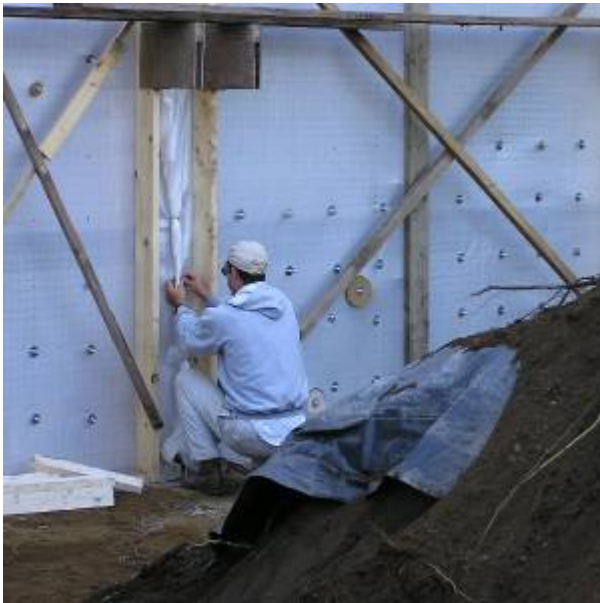
Wall Form Placement
