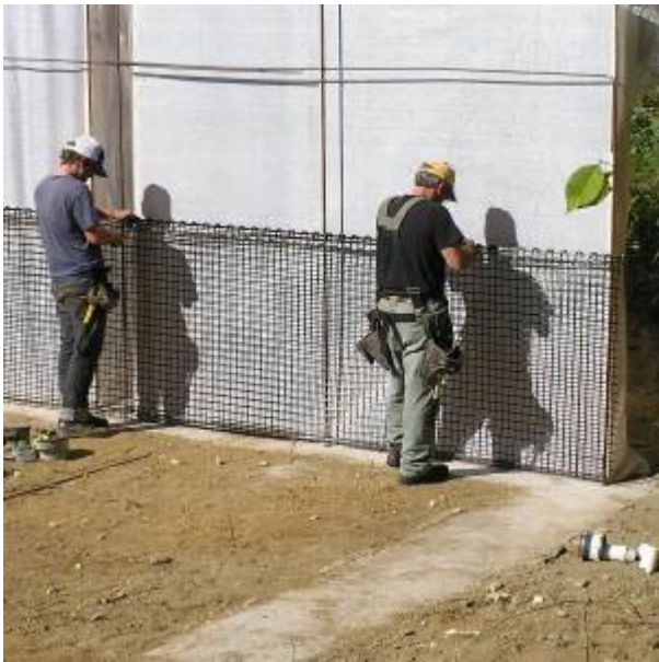
Adding Carbon Fiber Grid
