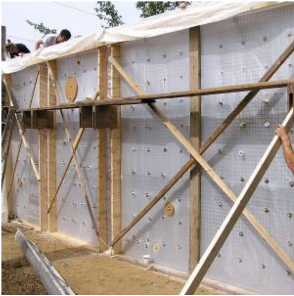
Wall Form Placement
