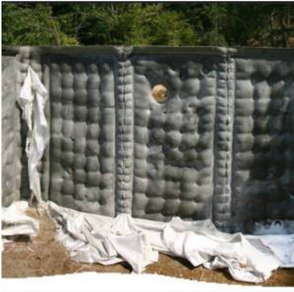
Stripping Formwork
