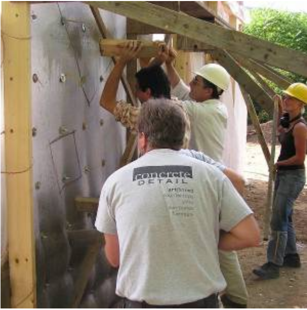
"Vibrating" Concrete
