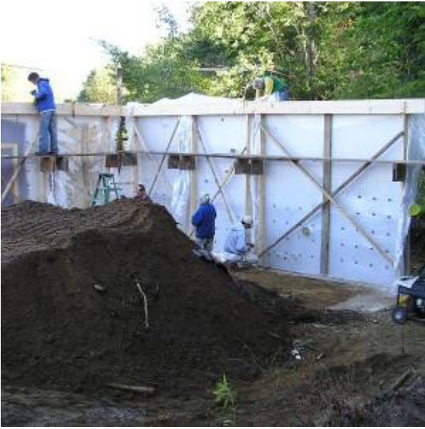
Wall Form Placement
