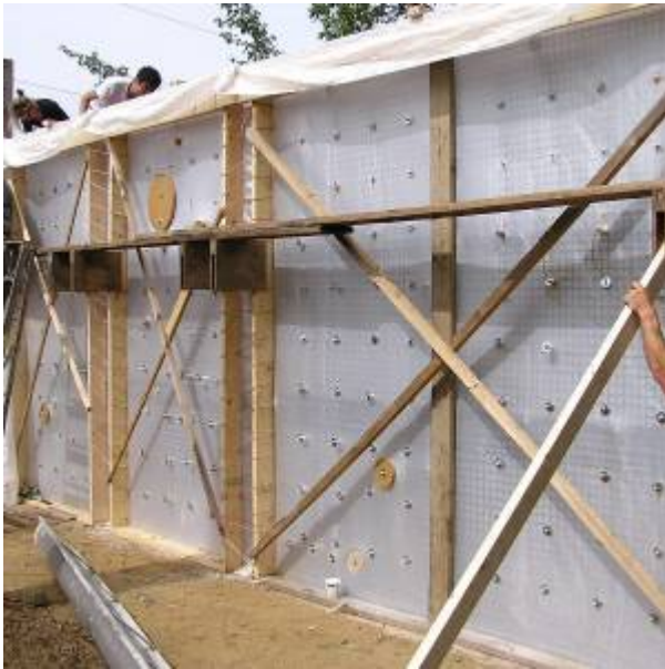
Wall Form Placement
