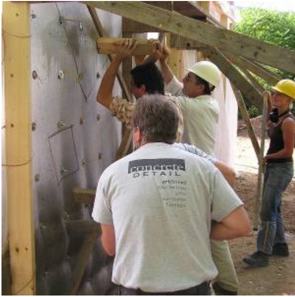
"Vibrating" Concrete
