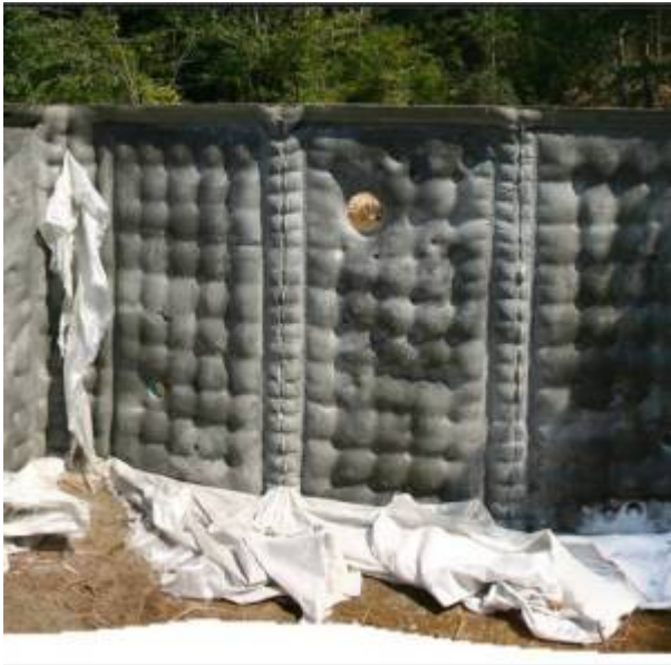
Stripping Formwork
