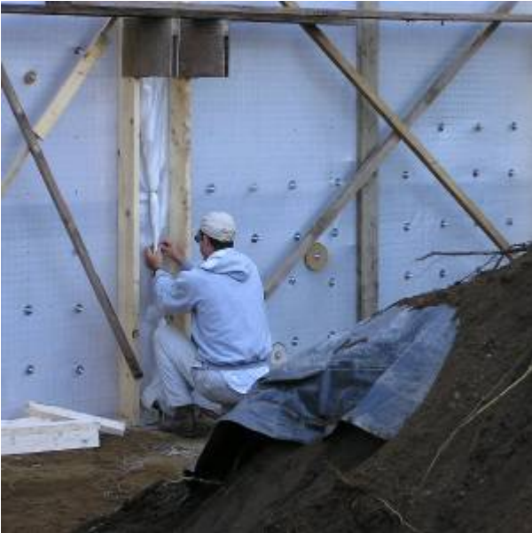
Wall Form Placement
