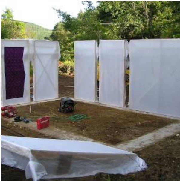
Wall Form Placement
