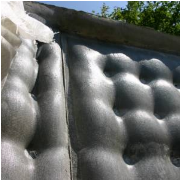
Stripping Formwork
