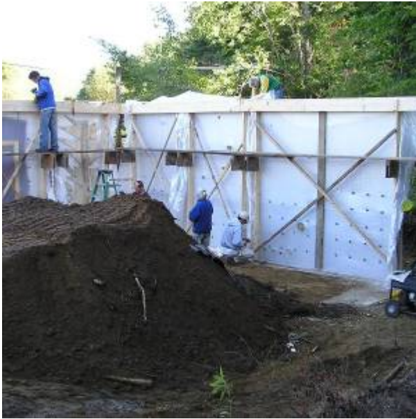
Wall Form Placement
