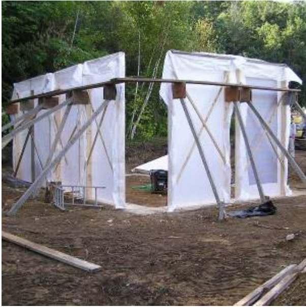
Wall Form Placement
