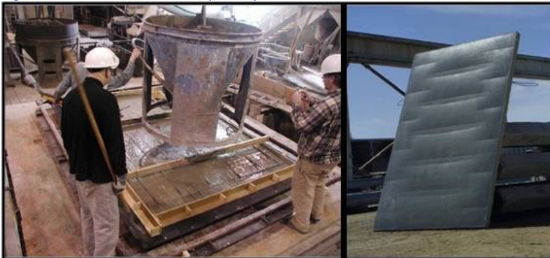
Fig. 2. Full-scale formwork and completed concrete panel.
