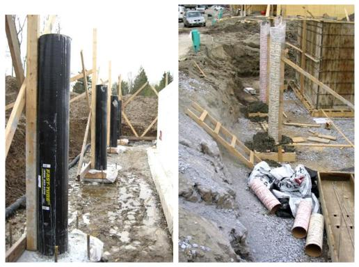
Figure A1: Commercially available column fabric formwork called Fast-Tube<sup>™</sup> (left) and conventional cardboard formworks (right) on a job site
