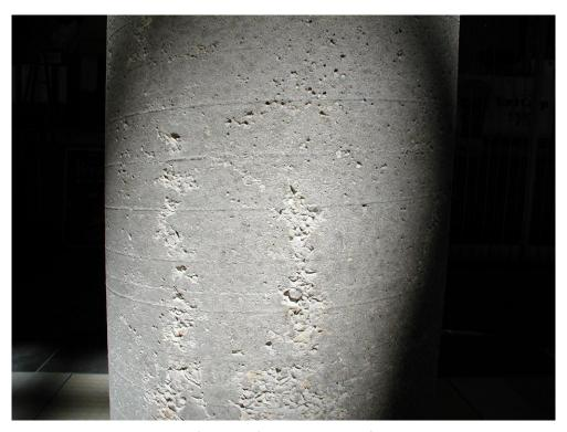
Figure 2: Bug holes and imperfections of a conventionally formed concrete column
