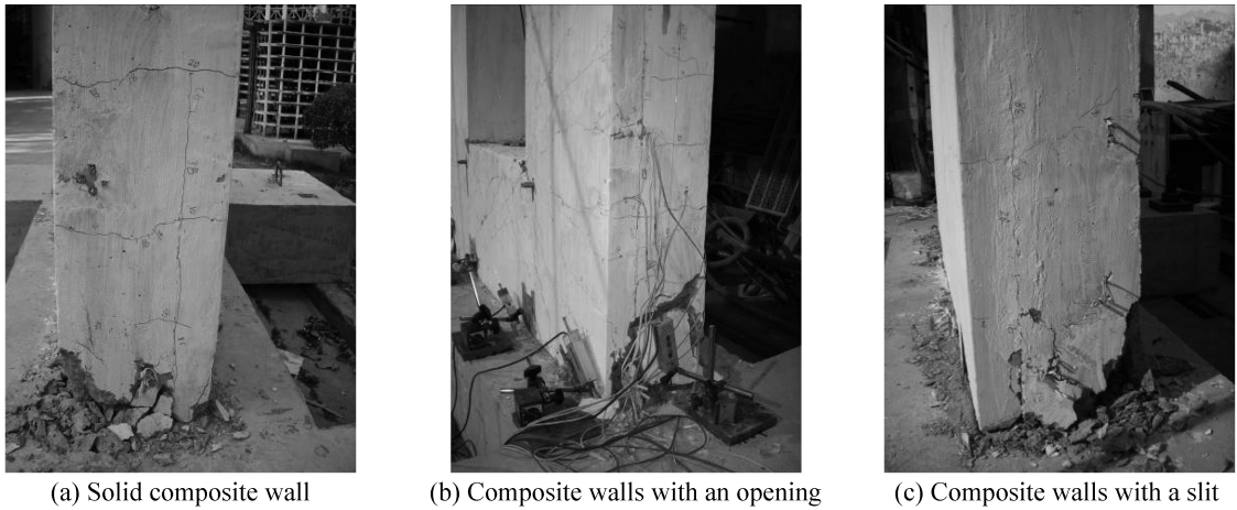
Fig. 12 Crack distribution at the edge of the specimens
