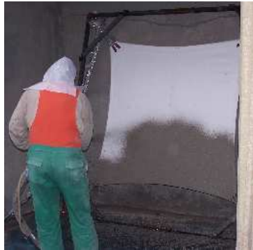
Figures 6 and 7: Applying the shotcrete to a pre-stressed PVC membrane.
