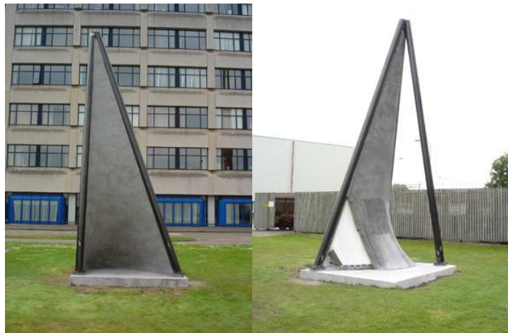
Figures 21 and 22: Back and front view of created concrete shell
