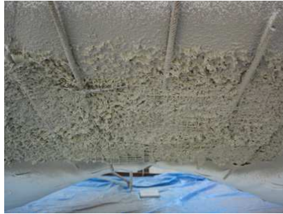
Figure 9: Shotcrete and reinforcement steel at the underside of a membrane
