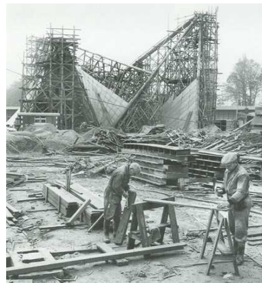
Figure 11: assembly panels on location
