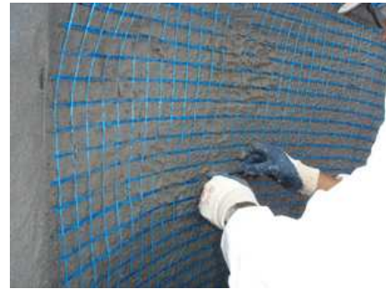
Figure 19: Shooting concrete on the membrane Figure 20: Applying the glass fibre netting
