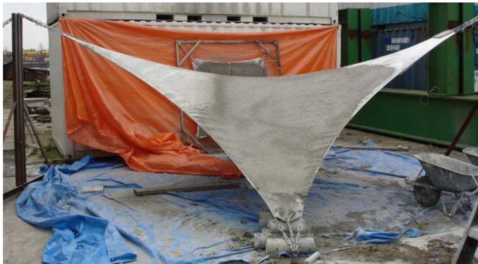
Figure 8: shotcrete on a double curved pre-stressed PVC membrane
