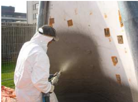
Figure 19: Shooting concrete on the membrane Figure 20: Applying the glass fibre netting
