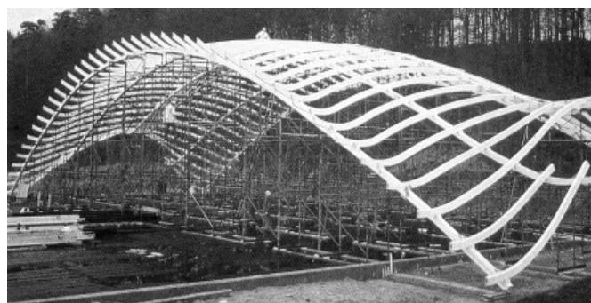
5-1: Linear support in a free form formwork [b]
