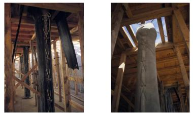
Figure 15: Fabric column formwork awaiting concrete placement (left) and column after cast
