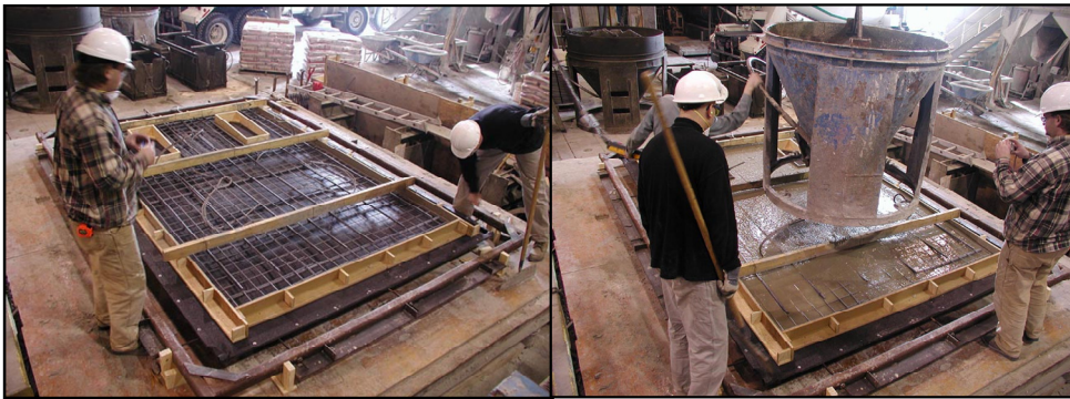
Figure 4: Securing fabric, reinforcement and pouring concrete in full-scale panel. (C.A.S.T. photos).
