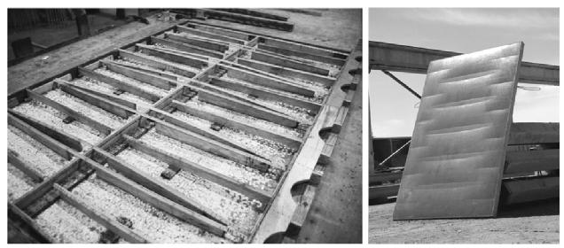
Figure 4. Full-scale formwork and completed concrete wall panel (C.A.S.T. photos).
