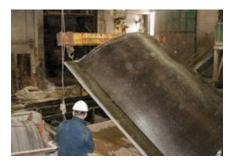
Fig. 16. Step 3 – Resulting funicular shell is inverted to form mold (C.A.S.T. photo)
