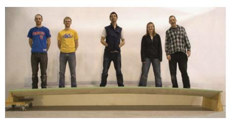
Fig. 21. Completed double curvature funicular thin shell vault (C.A.S.T. photo)
