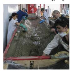
Fig. 20. Placing concrete and carbon grid in fabric mold to form double curvature funicular thin-shell vault (C.A.S.T. photo)
