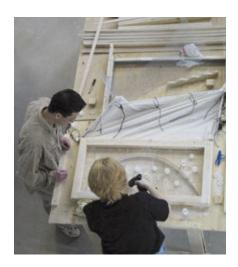
Fig. 6. Model wall panel formwork (C.A.S.T. photo)
