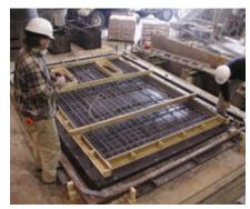
Fig. 9. Securing fabric and placing reinforcement in full scale wall panel formwork (C.A.S.T. photo)
