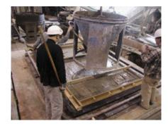
Fig. 10. Placing concrete in full scale wall panel formwork (C.A.S.T. photo)
