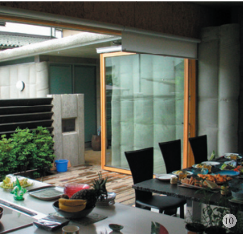
A flexible formwork membrane produces architectural and sculptural forms and surface textures as a direct result of construction decisions and details. The mold surface subtly changes its shape in response to the forces it resists.
