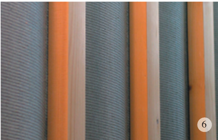
Fig. 6 shows a detail of an interior detail of a URC wall used in a commercial building by architect Shunji Kondo. Unno also acts as a consultant for other architects and builders wishing to use his URC formwork methods
