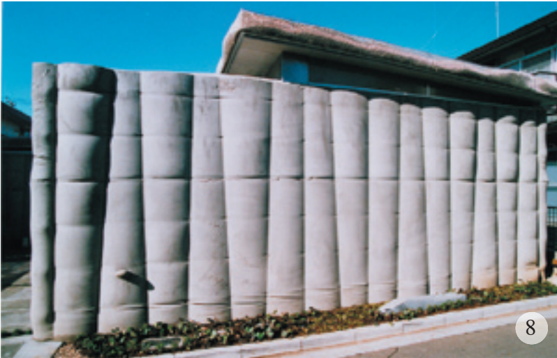
Fig. 8 shows the exterior concrete walls of Unno's "Stone renaissance" house, built in Funabashi City, Chiba for Susae Nakashima (2005). These walls are constructed using steel pipes restrained by standard form-ties running through holes drilled in the pipes. The (slightly diagonal) vertical impressions left by these pipes are freely composed as part of the wall's design.
