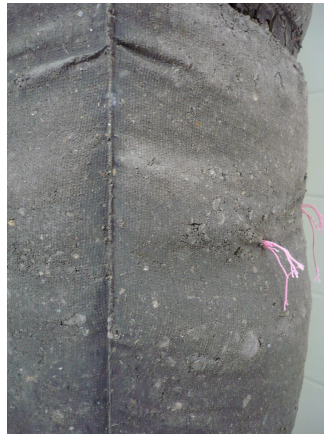
Figure 5: Detail of earth column with restraint thread visible 2007, image A. Chandler
