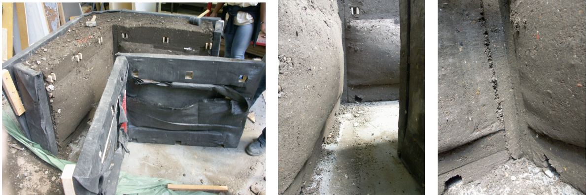
Figure 4: Climbing formwork strike and resulting earth detail, images A. Chandler
