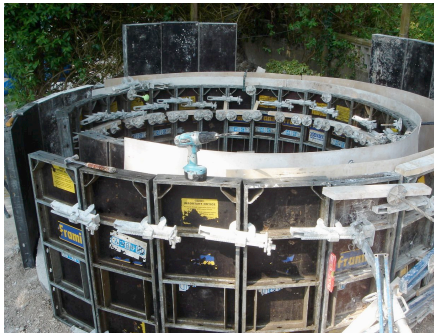
Figure 1: Concrete formwork for rammed chalk - Calyx visitor centre, Dover 2007 by Rowland Keable
