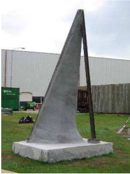
Fig.6, 7 The reconstruction of the red part of the Philips Pavilion by spraying shotcrete against a pre-stressed wire frame.
