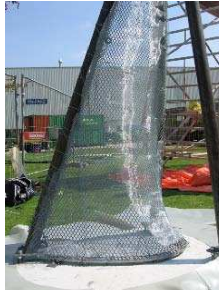
Fig.6, 7 The reconstruction of the red part of the Philips Pavilion by spraying shotcrete against a pre-stressed wire frame.
