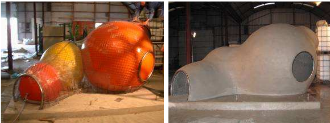
Fig. 1, 2 Blob structure rigidised with shotcrete.
