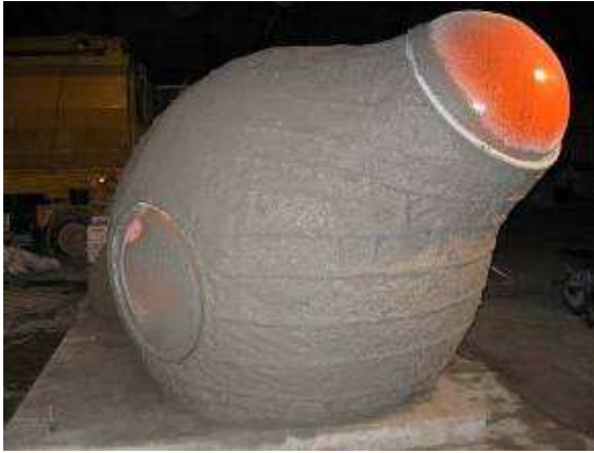
Fig. 16 Spraying the first layer of shotcrete .
