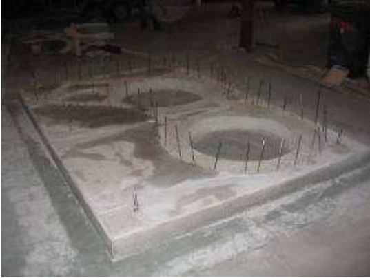
Fig. 13 The foundation of the prototype blob.
