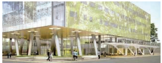
Figure 6: Entrance of the Women and Newborn Hospital, with a fabric-formed canopy (right).
