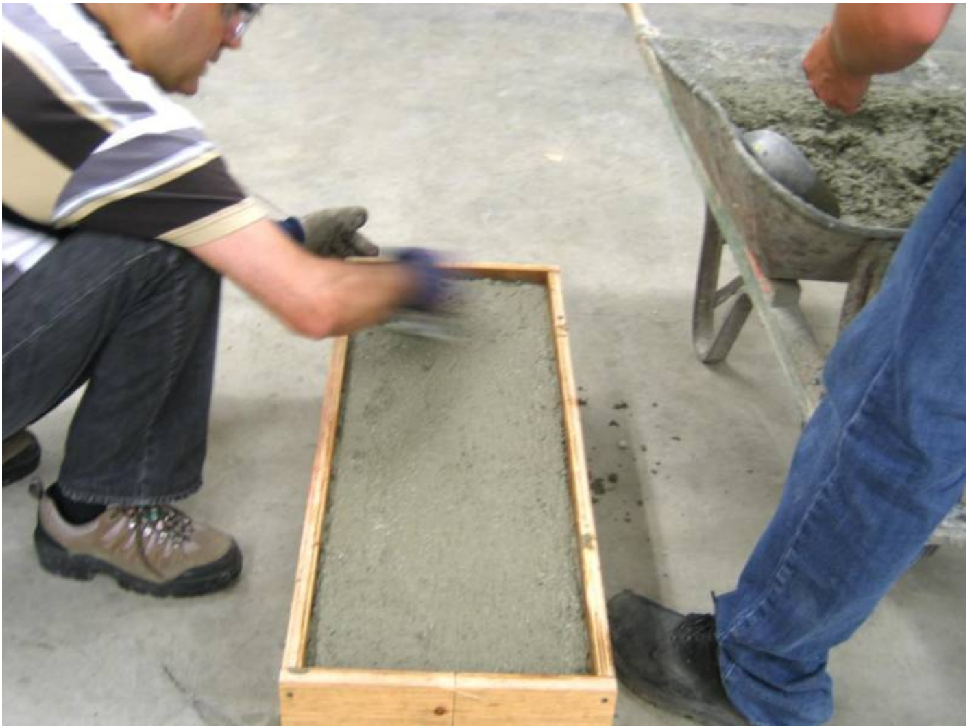
Figure 9: Filling the box with fresh concrete.
