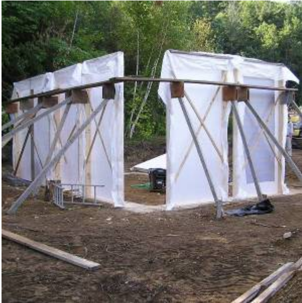
Fig. 5. Wall Form Placement
