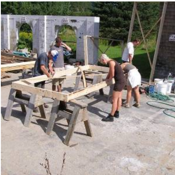
Fig. 1. Wall Form Assembly
