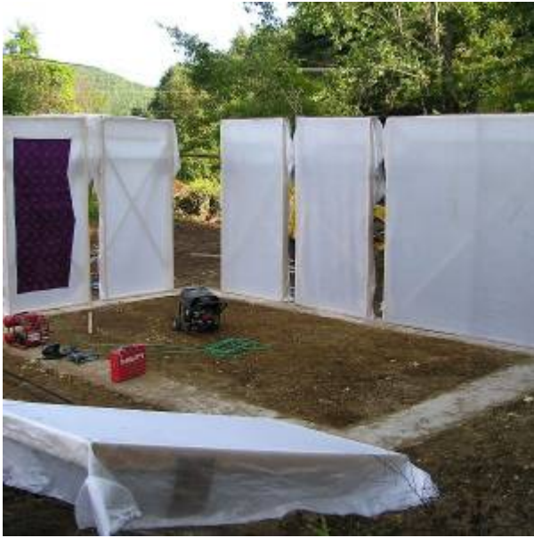
Fig. 4. Wall Form Placement
