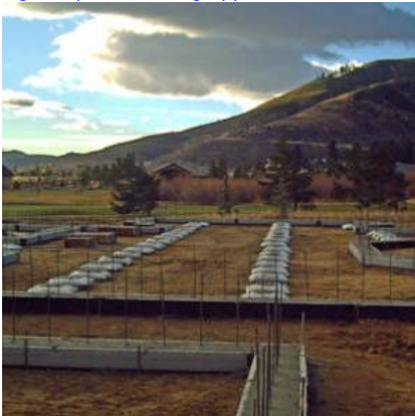
Fig. 4. Spread Footing Application
