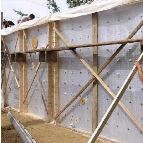
Fig. 8. Wall Form Placement
