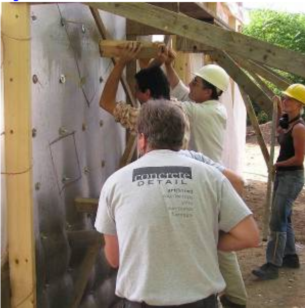
Fig. 11. "Vibrating" Concrete
